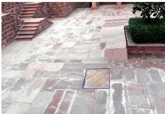
Entrance for manual O&M of second sedimentation tank
