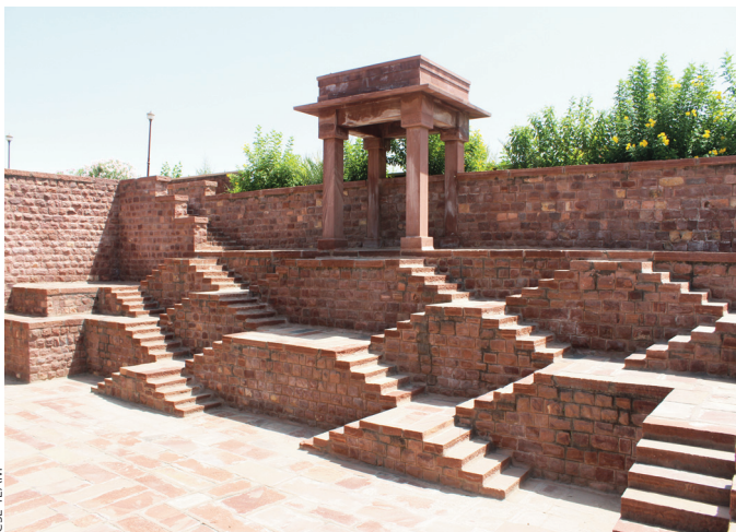
Entrance foyer similar to 'Kund'
