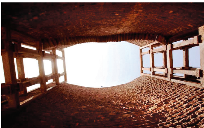
Vaulted walls for tank construction
