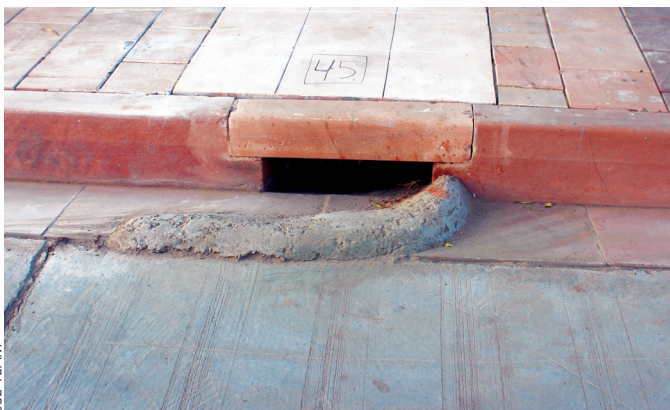
Inlet for road side drainage
