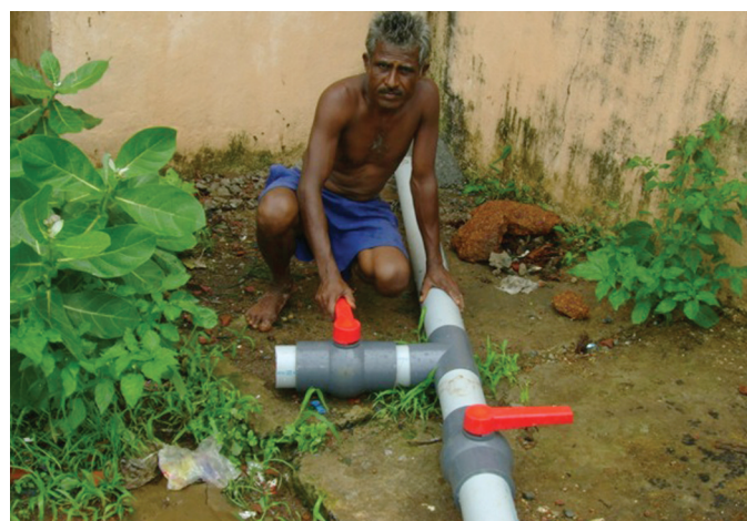
First flush device in use in the roof top RWH site on campus
